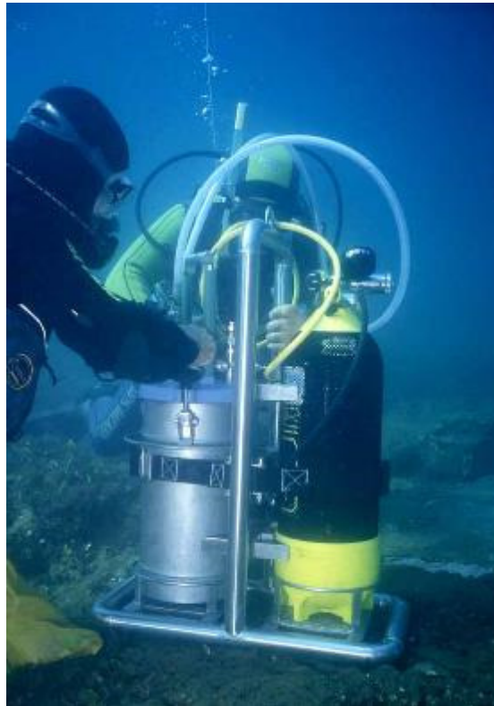
Figures 40 & 41. Manual joint and cracks filling (left) and with the use of an air compressed distributor (right). ©MiBACT-ISCR
