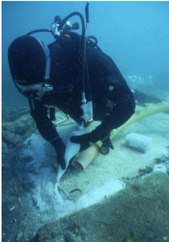
Figures 40 & 41. Manual joint and cracks filling (left) and with the use of an air compressed distributor (right). ©MiBACT-ISCR
