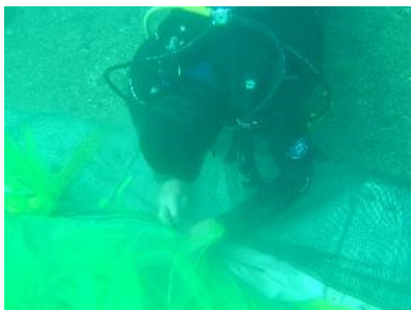
Figures 42 & 43. Manual joint and cracks filling (left) and with the use of an air compressed distributor (right).
